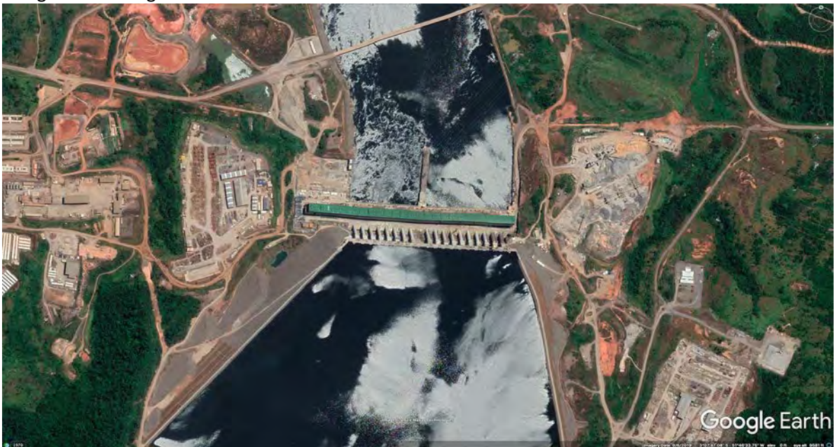
Google Earth image of the Belo Monte dam in 2019.
