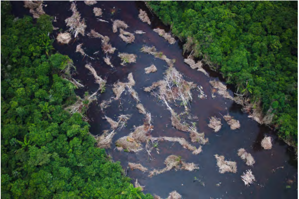
Dead trees in a canal constructed for the Belo Monte Dam project, near Altamira. Credit line: © Daniel Beltrá / Greenpeace
