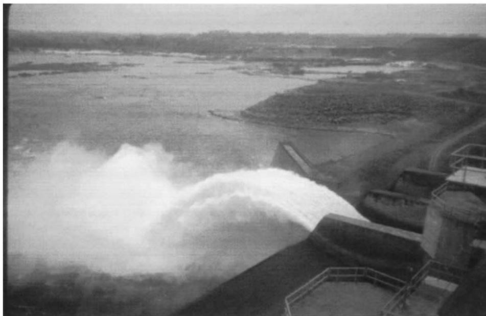
*Figure 2.* Spillway at Tucuruí. The ski-jump design oxygenates the water, but at the same time releases methane immediately. The spillway draws water from a depth of 20 m, where methane concentration is high (Fearnside, 2001).
