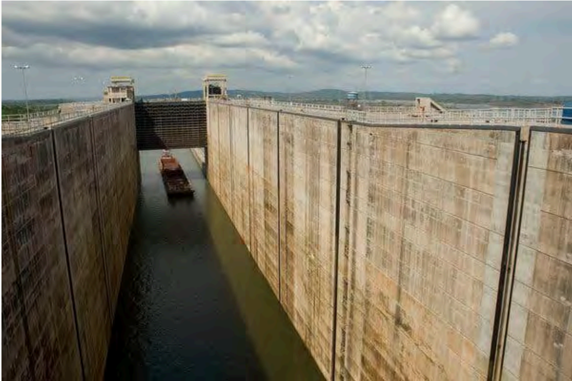
A barge navigating a lock of the Tucuruí Dam. Credit...Paulo Santos/Reuters
